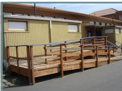
Inaccessible handrails on ramp
